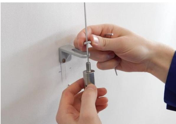
6. Install façade tightener to the bracket.
