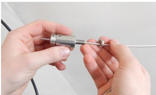
5. Put cable through façade tightener.
