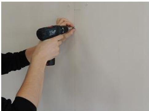
2. Drill holes, then mount brass clips using appropriate fixing system. Clips should be mounted along vertical axis
