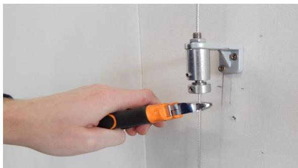
9. Cut out the excess of the cable.
