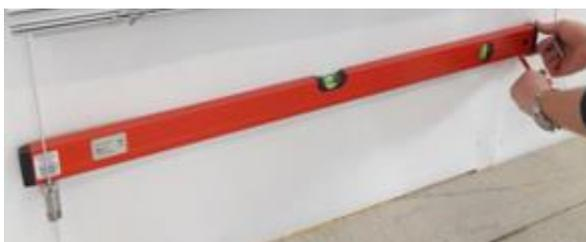
10. With a spirit level mark the installation place of the second cable guide bracket. Other actions perform analogically to the first bracket and guide.
