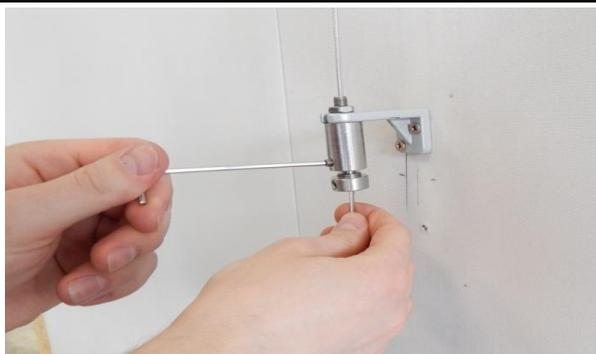
8. Loosen upper screw (locking movable part of the tightener). Stop when the movable part pulls out.
